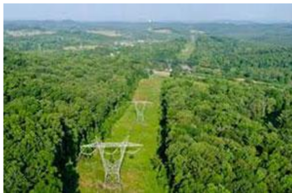
Electric utility right-of-way (Photo: www.jobs.tva.com )
