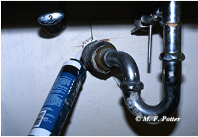
Fig. 9: Sealing around plumbing pipes helps reduce cockroach movement between apartments.
