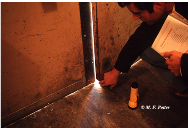
Fig. 3: Gaps under doors are a common entry point for spiders.
